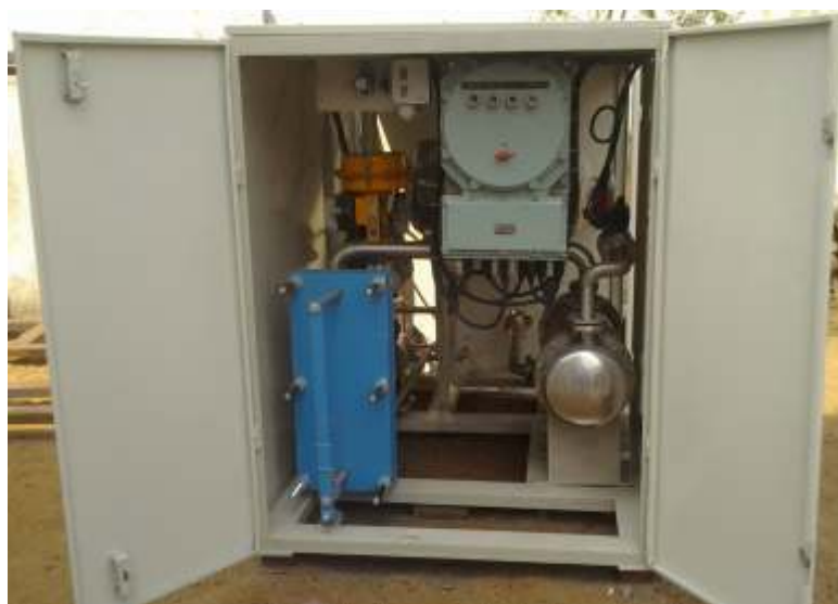
Above: Single Fluid Heating & Cooling System to accurately manage the temperature of the RCVD jacket.
